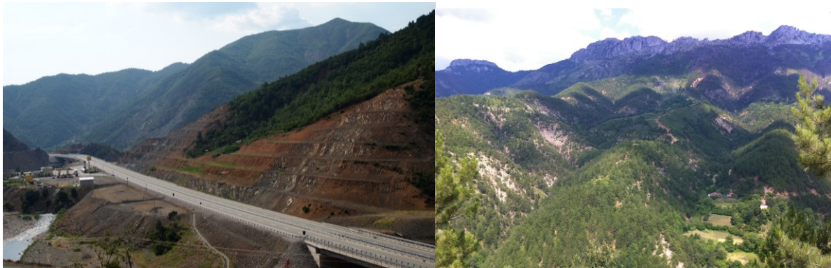
Figure 7: On the left: Fani i Vogel Valley, and the highway Durës/Kosovo. On the right: the village of Gryk, in the municipality of Orosh.
