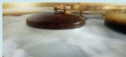
Figure 176 - Water pressure dissipation using a load breaker
