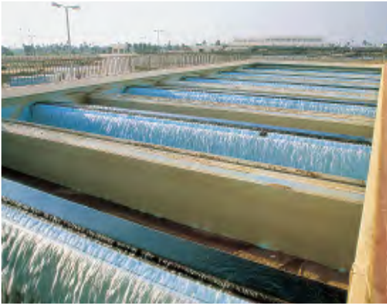
Figure 2: Water treatment plant.
